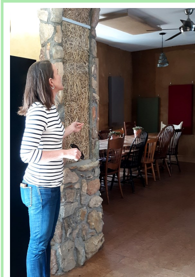
Inside the straw bale building, O'Herron points out a section where customers can view the interior of the building filled with straw.
